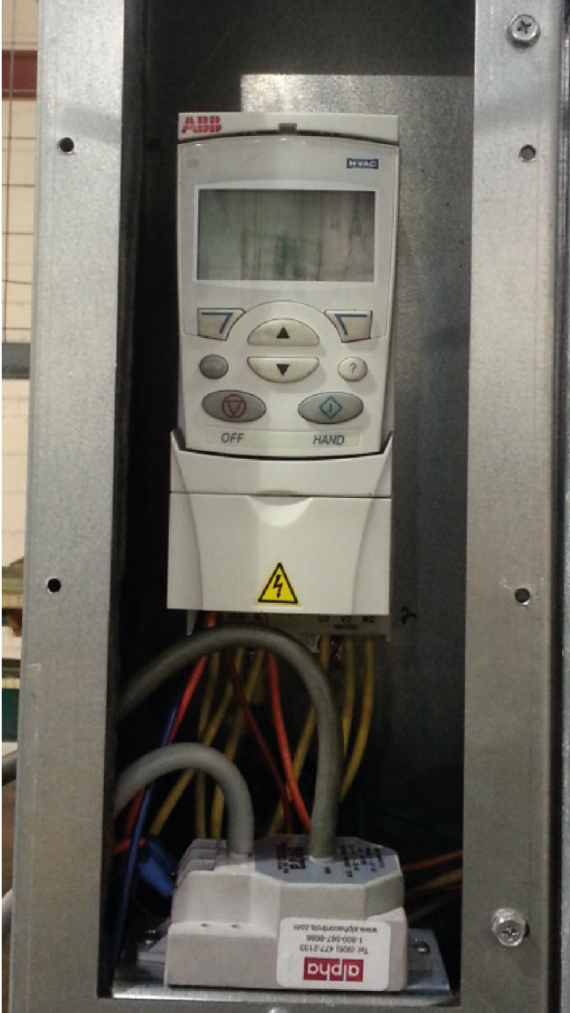
Figure 4: VFD keypad and Ethernet connector (CSV/DSH shown)
