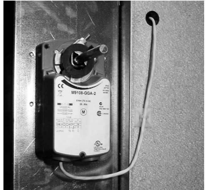
FIGURE 10 - SECURE CABLE WITH ROUTING HARDWARE
