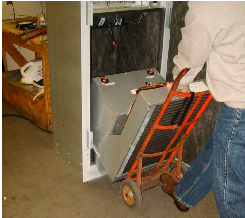
Figure 27: Insert the chassis
