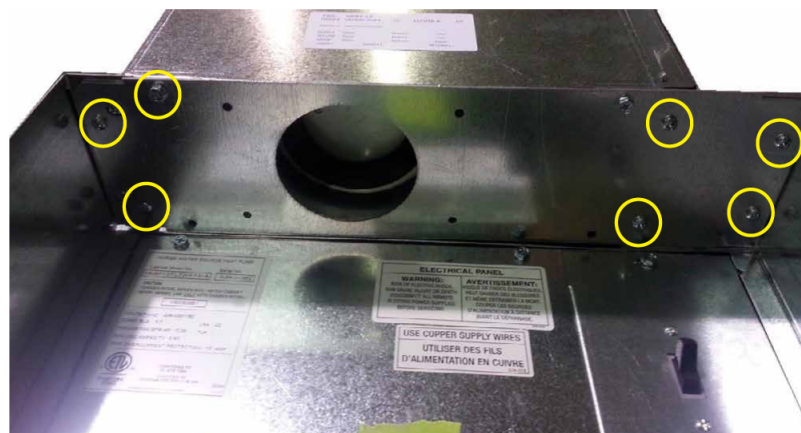
Figure 19: Damper plate fasteners
